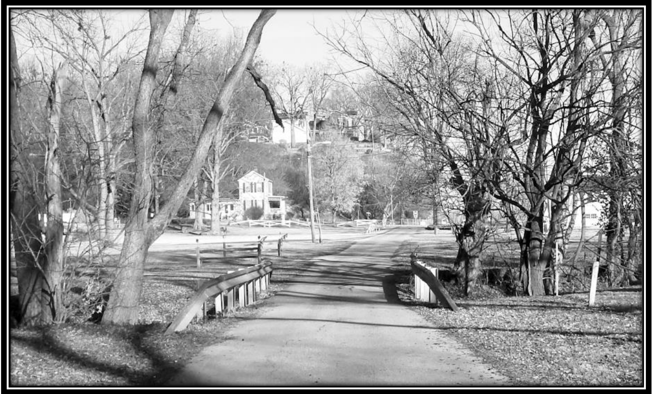
A December, 2019 photo of the bridge on First Street over Spanker's Branch looking north to the bluff.
